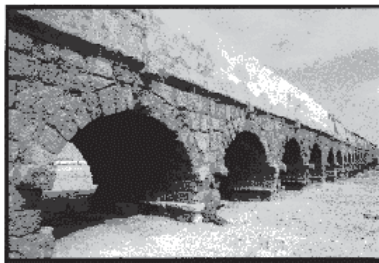
A Roman aqueduct
